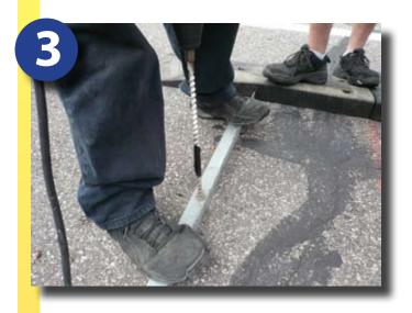
Be careful to prevent any movement of the steel bars once they are positioned. With the corner modules still in place, drill through the holes in the bars to a 4-inch depth.
