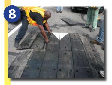
Once the steel bars are secured to the road, fit the ramps on the steel. Be sure to position the arrows in the direction of vehicle approach. Tap the modules on the sides with a hammer to make them fit snugly and align properly.
