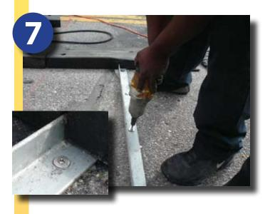
Using the impact wrench with the T40 torx bit, carefully drive the torx lag bolt so it is snug to the steel (see inset). **Do not overtighten.** Clean up any excess resin from around the bolt with a rag.
