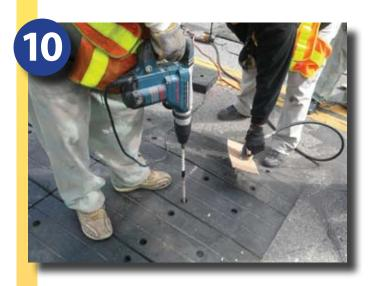
Blow the drilled holes clean with the long-nose air nozzle. Drilling and cleaning holes can be done at the same time.
