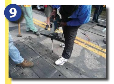
Drill all the holes to a depth of seven inches from the *top* surface of the module.
