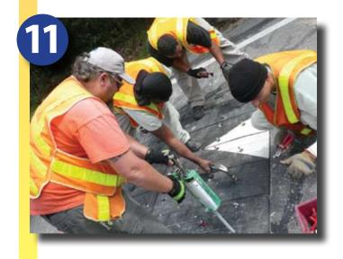
Inject one pump of resin into each drilled and cleaned hole and insert lag bolt immediately. Tap the bolt into the hole so the RediPlug is at full depth and the anchor bolt is about 1 1/2 to 2 inches above the surface of the module. Tighten the bolt with the impact wrench until the washer is snugly seated. **Do not overtighten.**
