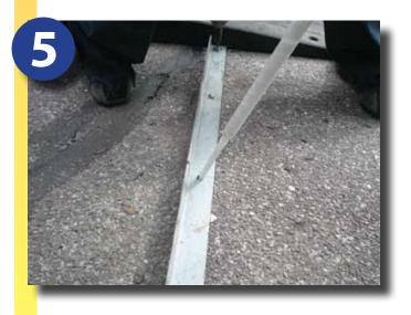
Inject one pump of resin into each drilled and cleaned hole. The resin will dry quickly, which is the reason for extra nozzles.
