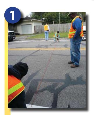
Measure and mark the correct position on the road for the cushion. Snap a chalk line across both lanes so the cushions can be properly aligned with each other across the road. Center each cushion within the lane, keeping in mind that this original placement will determine all other steps of the installation process. Typically, there should be no more than four feet between each cushion.
