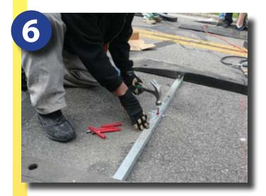
Gently tap the torx anchor assembly into the hole with a hammer to the point where the RediPlug is flush to the top of the hole.
