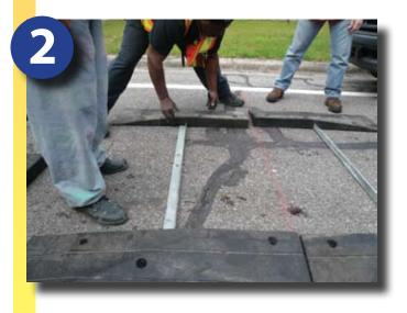
Place the four module corners on the steel bars, being sure they are squared and properly positioned according to the markings. Be certain the corners are snug against each other. This will determine the final position for the steel bars.
