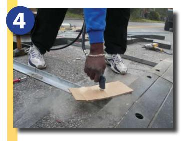
Using your long-nose air gun, blow all debris out of the holes.
